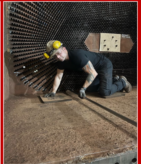
Andy Vansock installing the last tube at Brunner Island at 20:05
